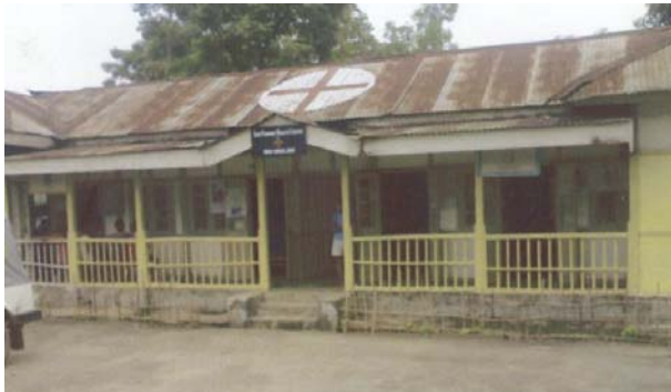
Primary Health Centre Tizit
