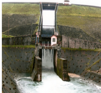
Anjunem Irrigation Project (AIP)
