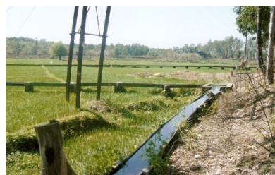
Field Channel in Command Area of Salaulim Irrigation Project
