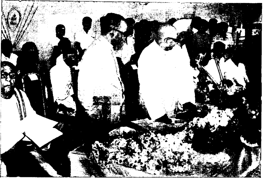
FERTILISER FOR INCREASED PRODUCTION—LAYING OF FOUNDATION OF THE RAMAGUNDAM FERTILISER PROJECT BY DR. TRIGUNA SEN, UNION MINISTER FOR PETROLEUM AND CHEMICALS ON 2ND OCTOBER, 1970
