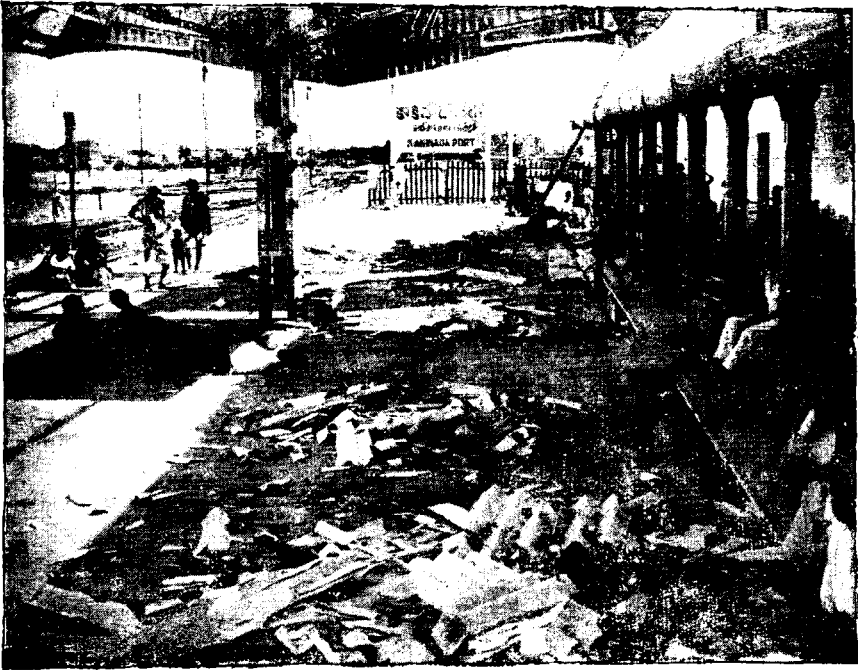
“THE DESTRUCTIVE FORCES OF NATURE AT WORK” BATTERED KAKINADA PORT RAILWAY STATION
