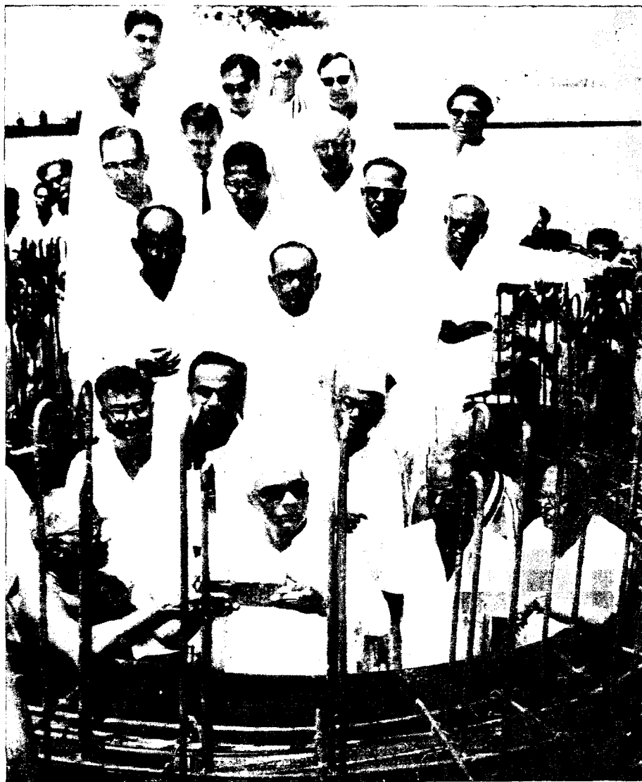
LAYING OF FOUNDATION STONE FOR THE SIR ARTHUR [COTTON] BARRAGE BY THE HON'BLE CHIEF MINISTER OF A. P. ON 11-4-70. SEEN IN THE BACKGROUND IS THE OLD ANICUT "THE OLD ORDER CHANGETH YIELDING PLACE TO THE NEW".
