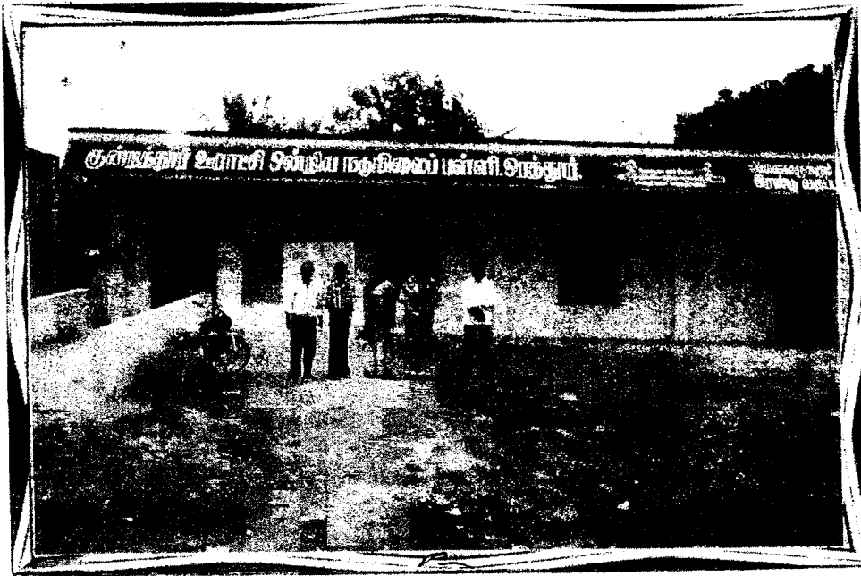
Community Construction – Two Classroom Building
