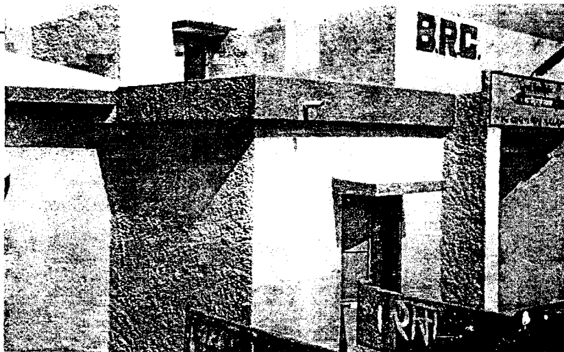
BRC BUILDING RAMTEK, DIST. NAGPUR
