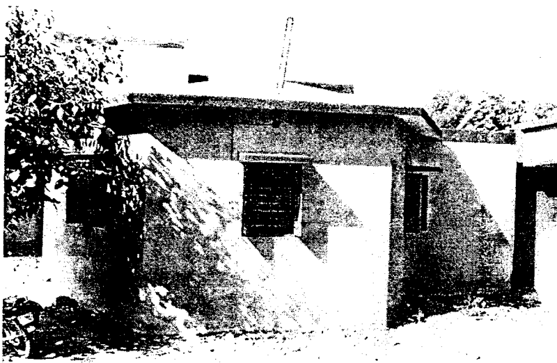
BRC BUILDING KAMTEE, DIST. NAGPUR
