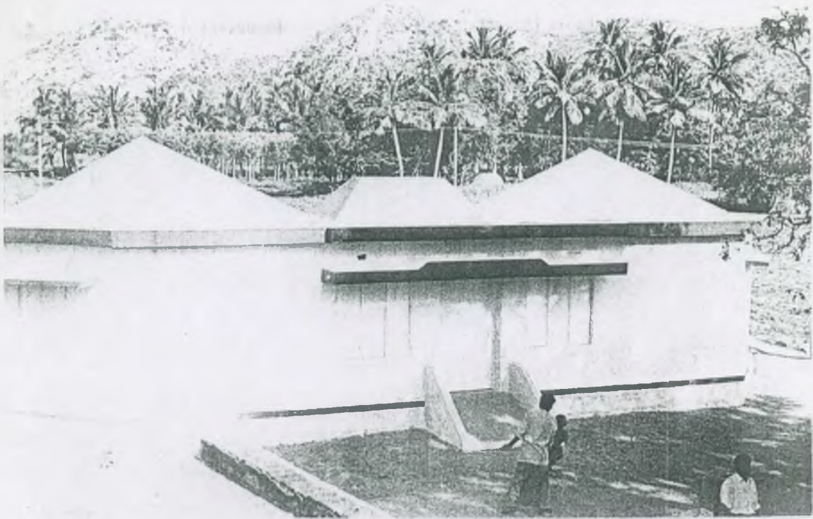
14. TWO CLASS ROOM BUILDING P.U.PS PERIASEMMETTUPATTI USILAMPATI BLOCK
