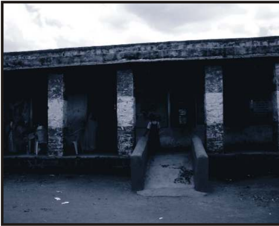
School Building with Ramp
