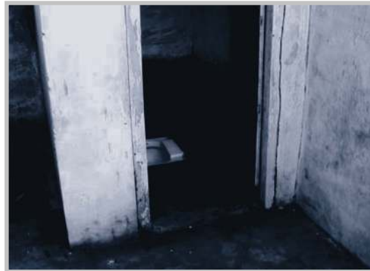
Toilet facility in Santhamarur School, Hassan Taluk
