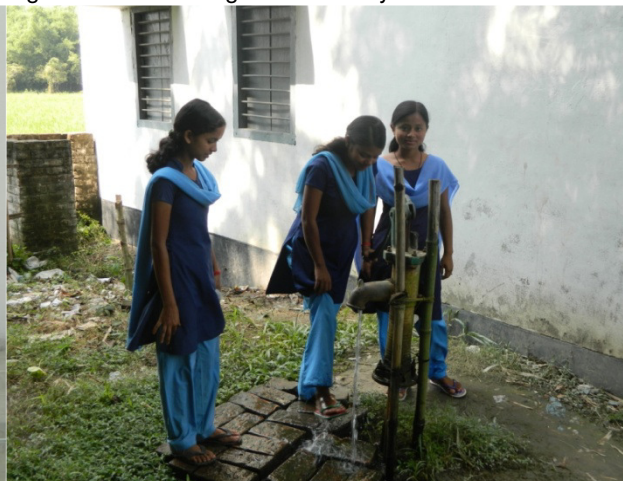
Figure 4.16: Drinking Water Facility in School
