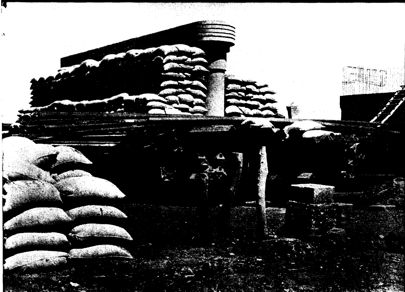
↑ TEST LOADING OF ONE OF THE PIERS OF THE UDDUTERI BRIDGE IN KRISHNA DISTRICT.
