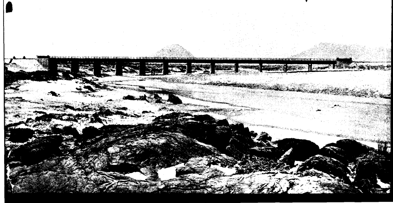
PILLAPERU BRIDGE ON THE KANIGIRI-BADVEL ROAD IN NELLORE DISTRICT. ↓
