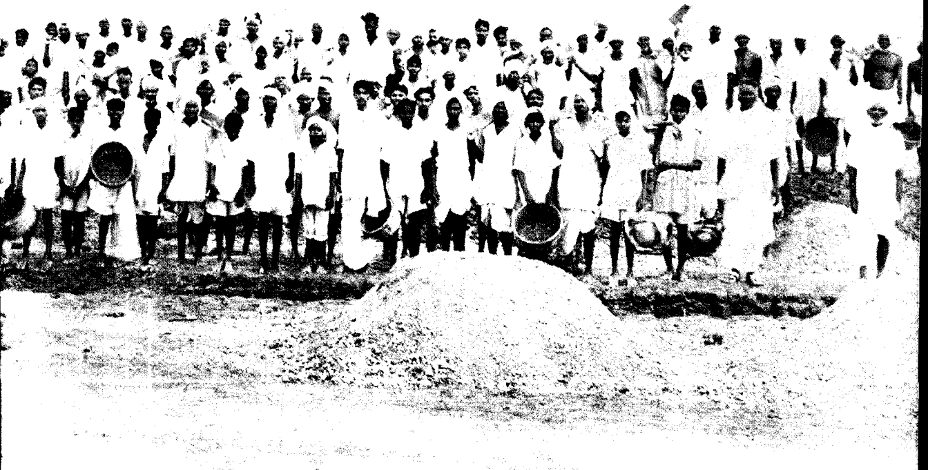
↑ ROAD WORK IN PUSAPADGI (BAPATLA TALUK) UNDER LOCAL DEVELOPMENT WORKS SCHEME.
