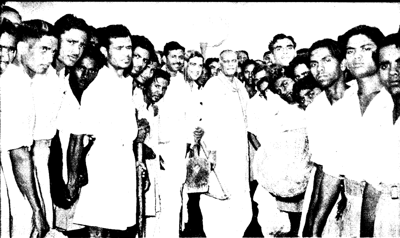
↑ THE PLANNING MINISTER WITH THE BHARAT SEVAK SAMAJ WORKERS DOING ROAD WORK IN NANDYAL.
