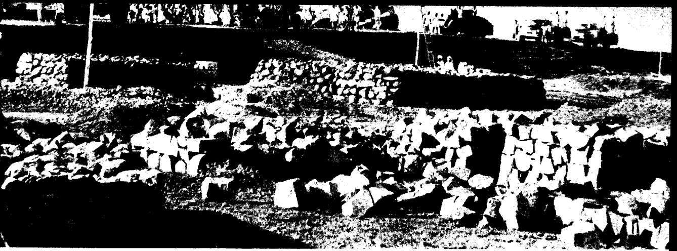
↑ A PANORAMIC VIEW OF THE LEFT FLANK EARTHEN BUND OF THE BHIRAVANTIPPA PROJECT
