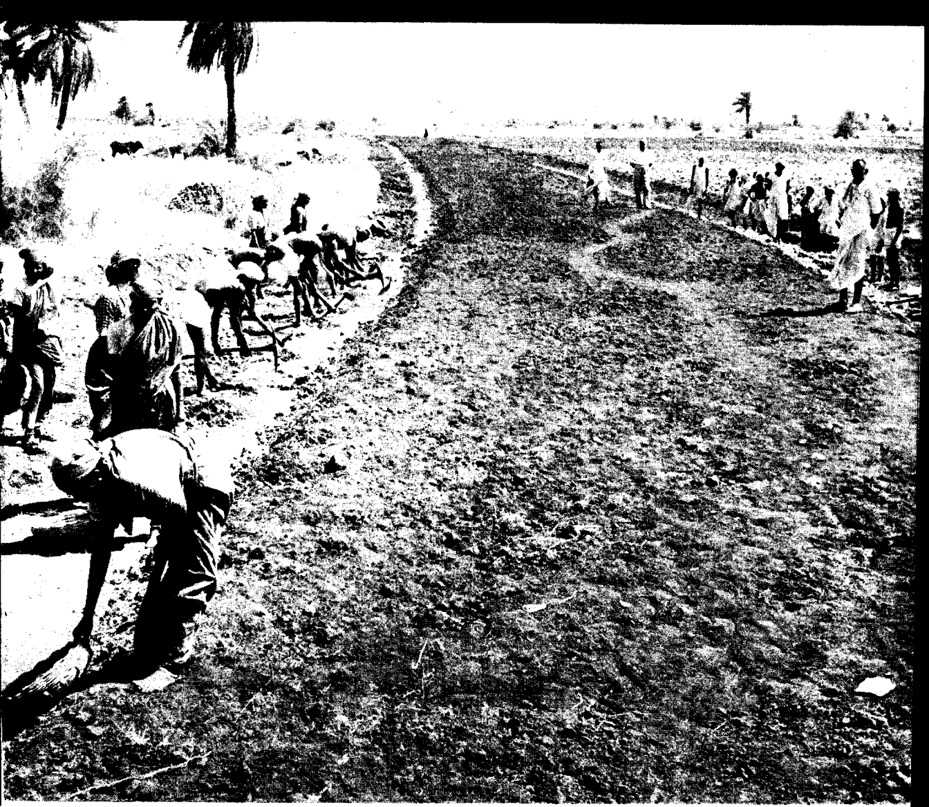
ROAD LAYING BY VILLAGERS IN KURNOOL-CUDDAPAH CANAL COMMUNITY PROJECT AREA.
