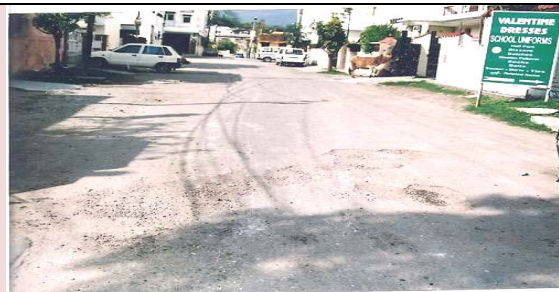
Picture: Repair of internal road in Vasant Vihar Enclave (Dehradun).
