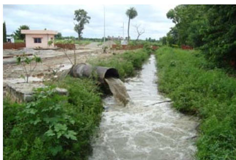
Pictures 15 & 16: The untreated sewage bye passing from STP draining directly into Ganga (July 2010)
