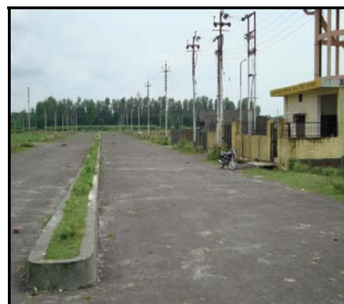
Picture 14: Laksar village road at Transport Nagar July 2010
