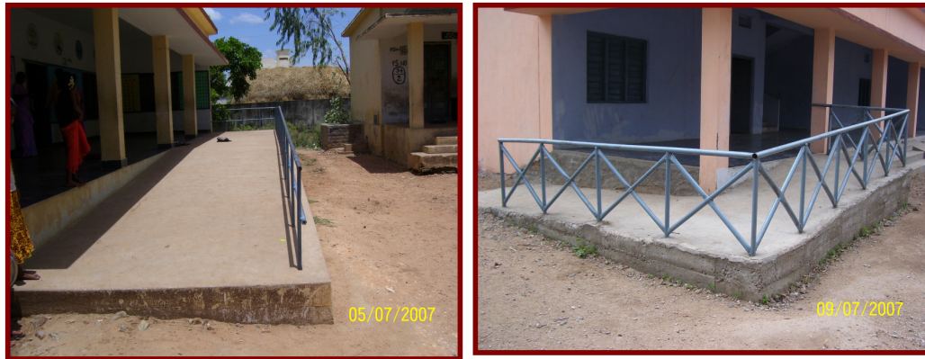
Ramps in different school buildings
