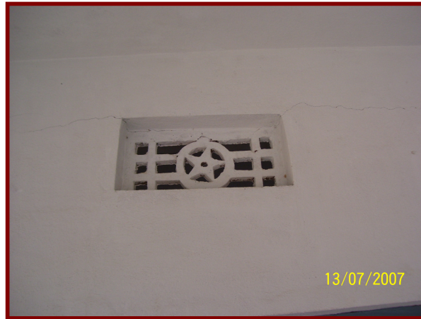
Ventilation and jalli work
