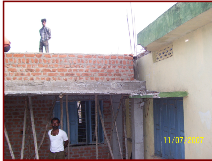
Synchronization of old building with new construction
