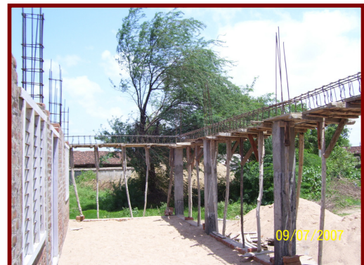
Shuttering in progress
