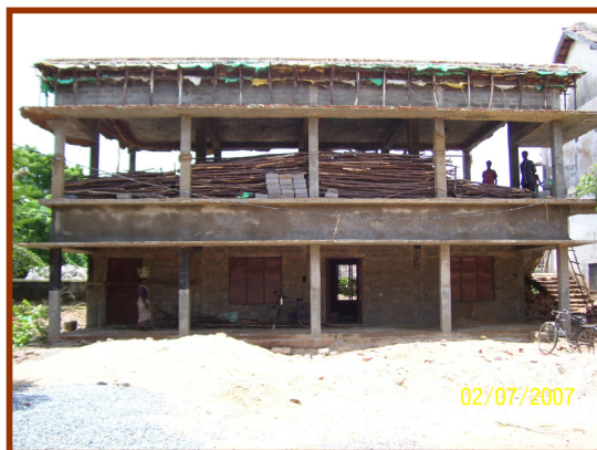
Building work in progress
