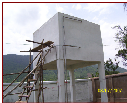
Drinking water storage tank
