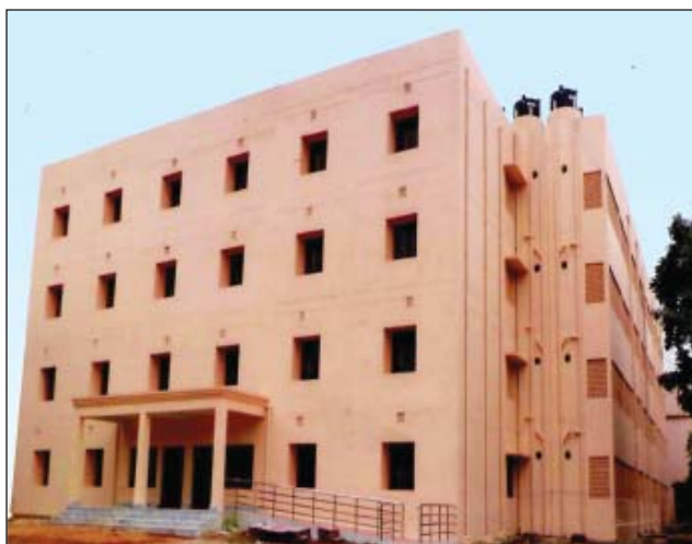
Hostel Complex at BJB College, Bhubaneswar
