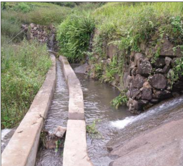
Construction of field channel at Darangia nala at Rudhei
