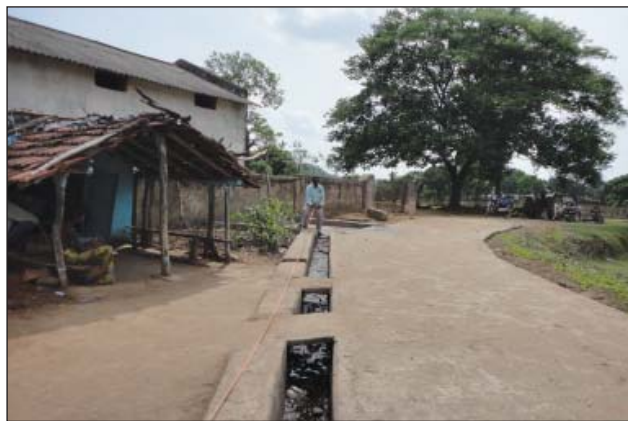
CC Road & Drain at Bamiring
