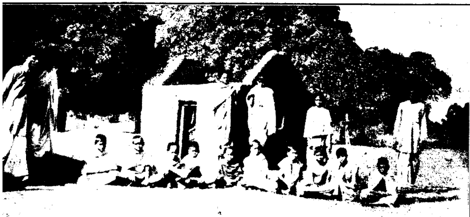
A VILLAGE SCHOOL IN ANGUL. MODEL HOUSE UNDER CONSTRUCTION.
