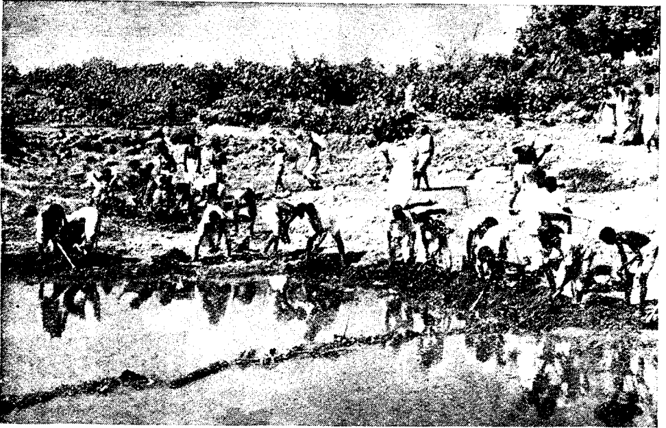
Cleaning a tank, Raneshwar.
