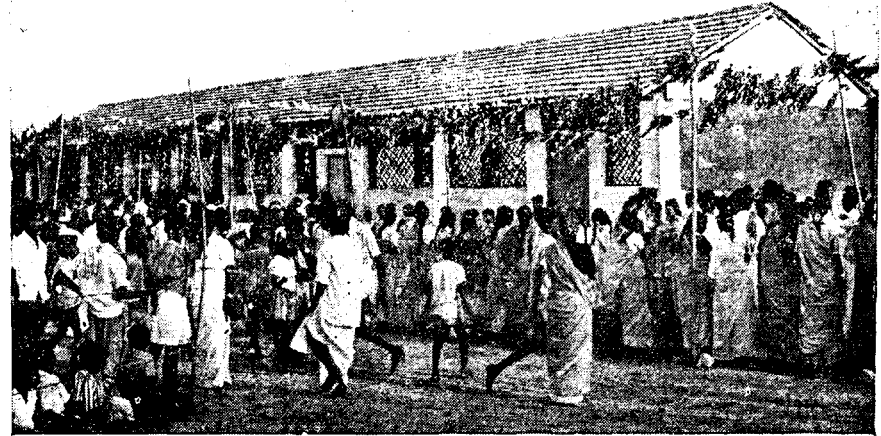
School Building Constructed at Urur Adyar by the Prosperity Brigade
