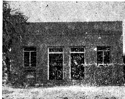
Headmaster's Office Room Constructed at G. H. S. Vettavalam.
