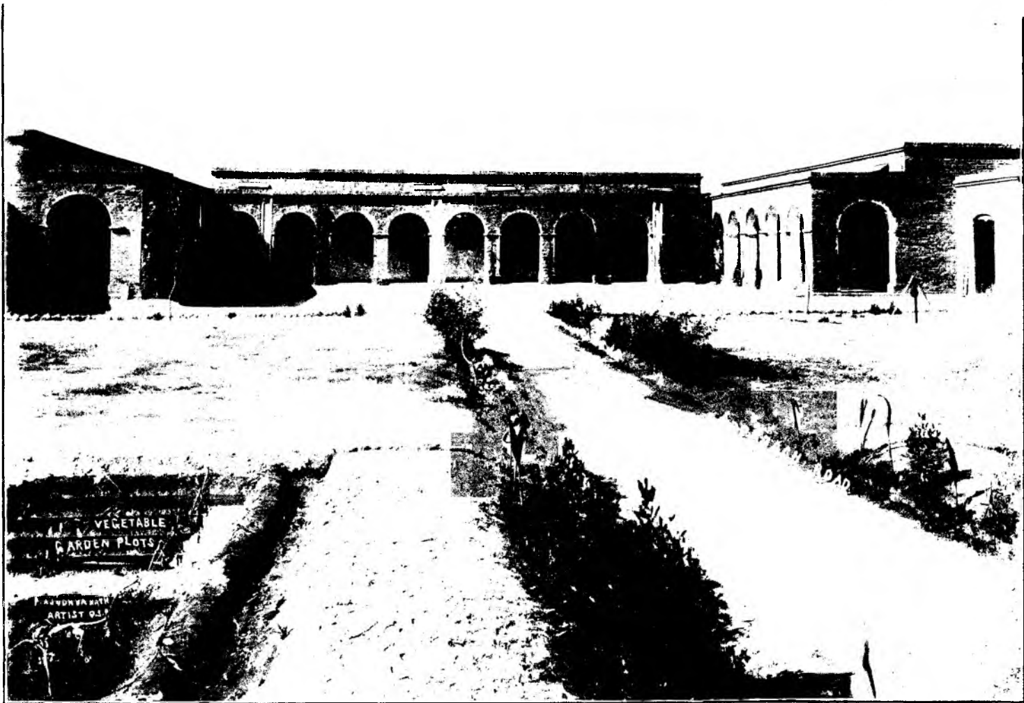
D. B. VERNACULAR MIDDLE SCHOOL, BURJATTARI, SHEIKHUPURA DISTRICT.
