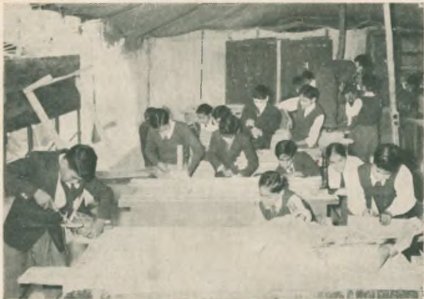
A carpentry class at work
