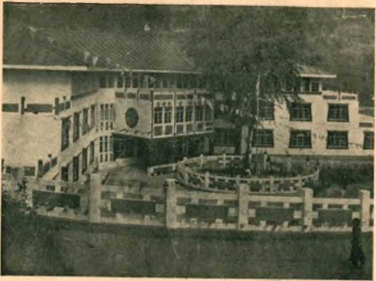
Newly constructed District Administration Centre at Namchi
