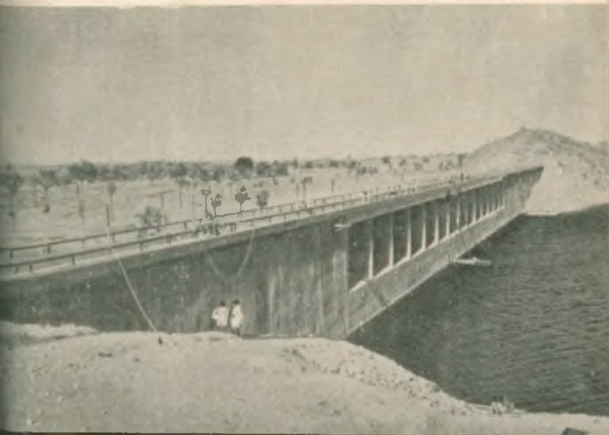
Tilaiye dam of D.V.C. : View of the dam from the river-side.
