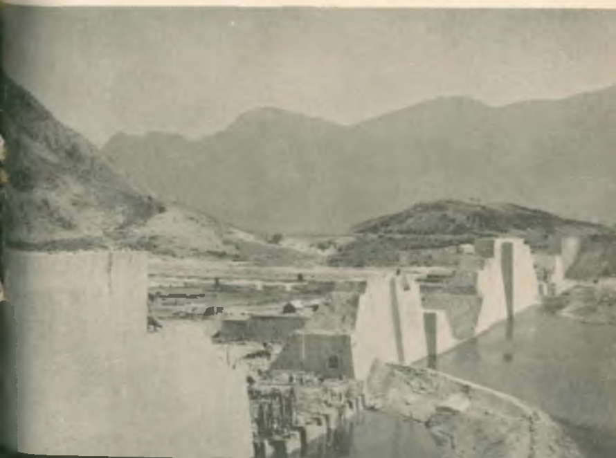
Malampuzha Project : A view of masonry dam.
