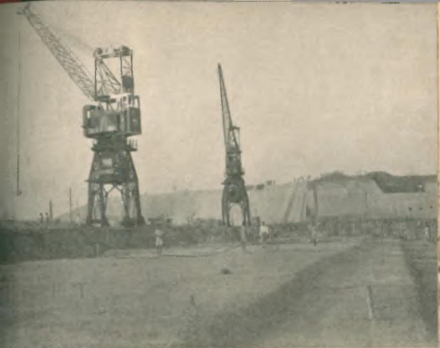
Hirakud Project : A view of the left concrete dam.
