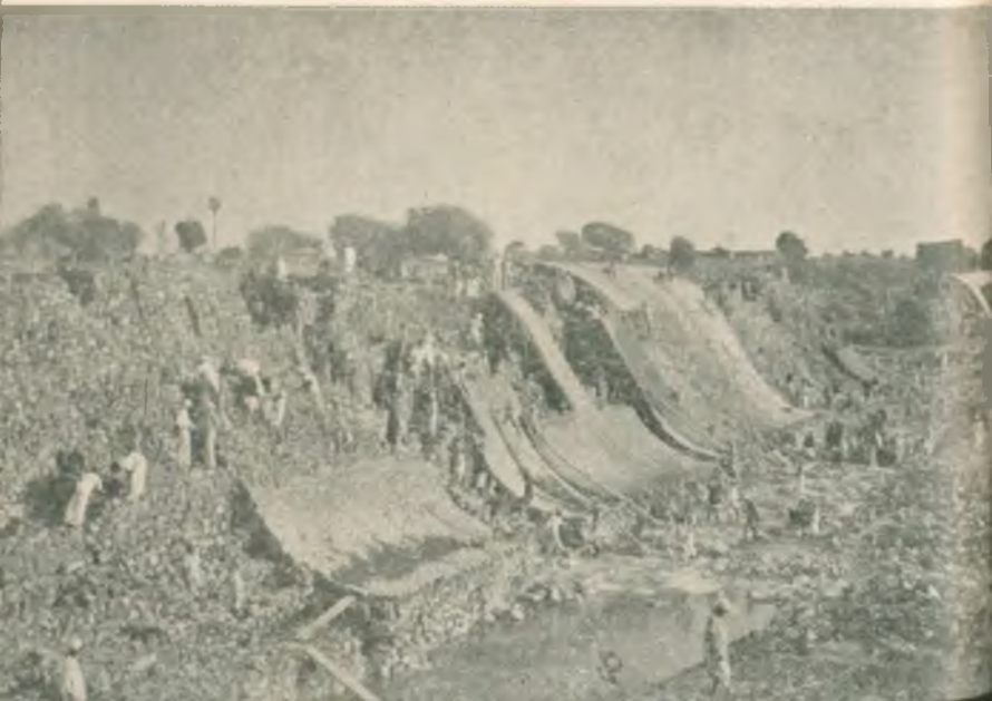
Kakrapar weir under construction.
