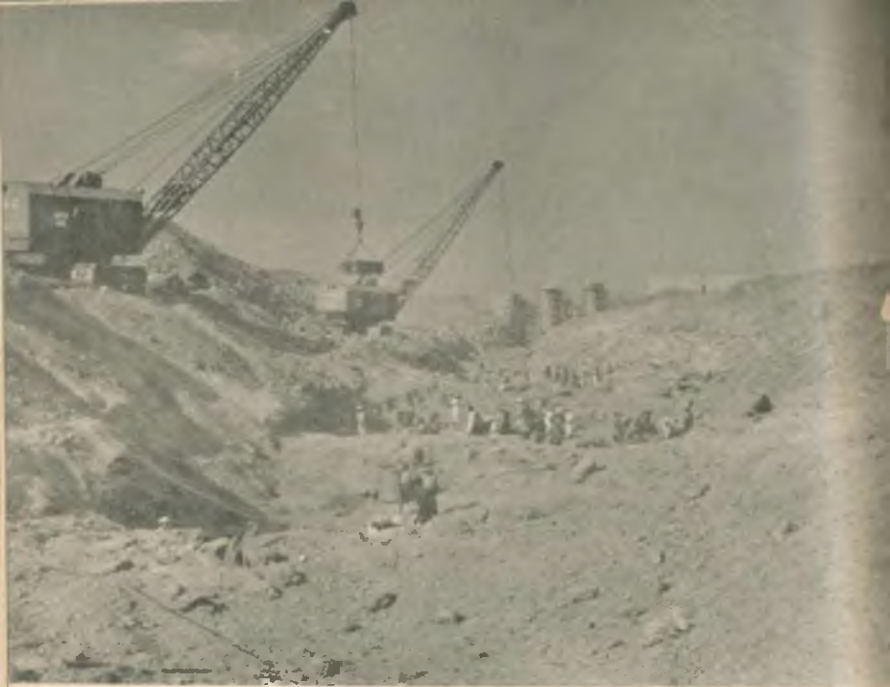
Kakrapar Project Gujerat : Excavation work is on.
