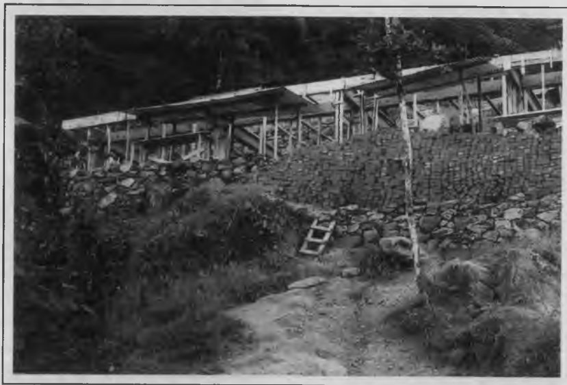
4 additional class room under construction -- .....
