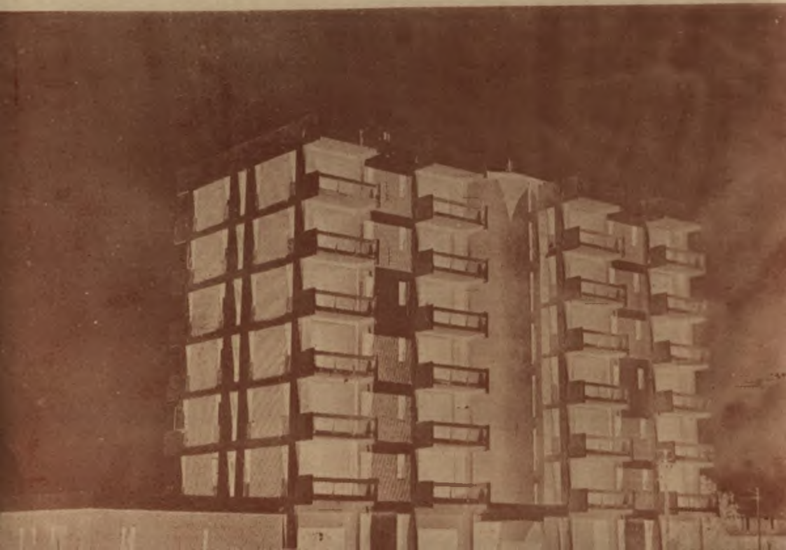
The hostel building under construction
