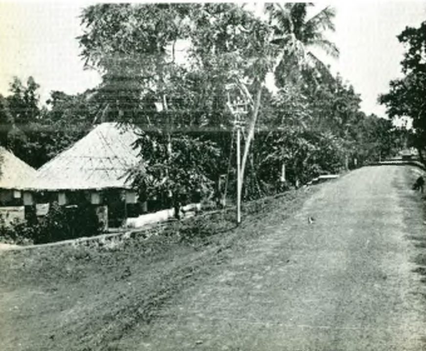
Ext. C/99 (4) Approach road of Post Office, embankment road in front of P. S., P S building and steps and urinal
