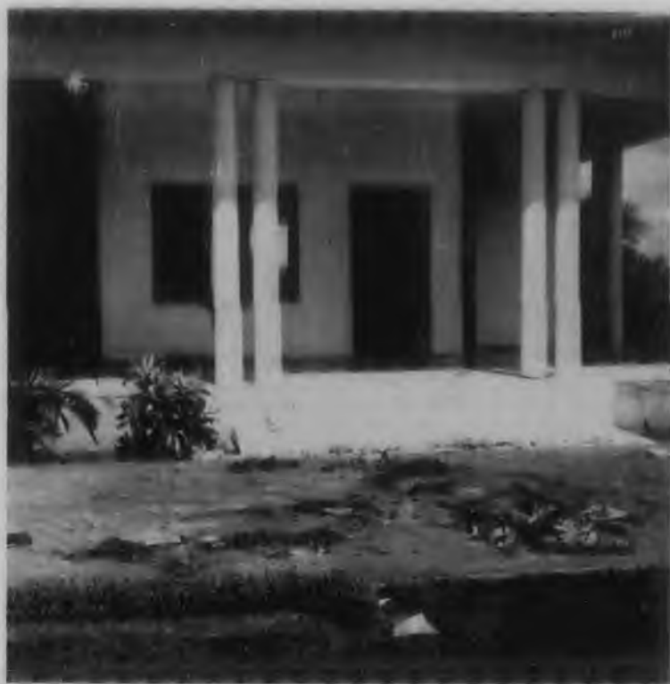
A scene showing the damaged and burnt articles lying in front of the residence of Shri B. Patnaik
