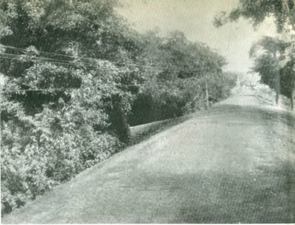
Ext. C/99 (3) Embankment road towards East and approach road
