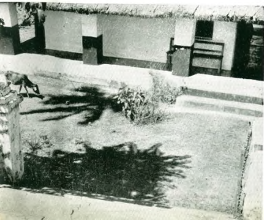
Ext. C/99 (6) Gate and some portion of P S building
