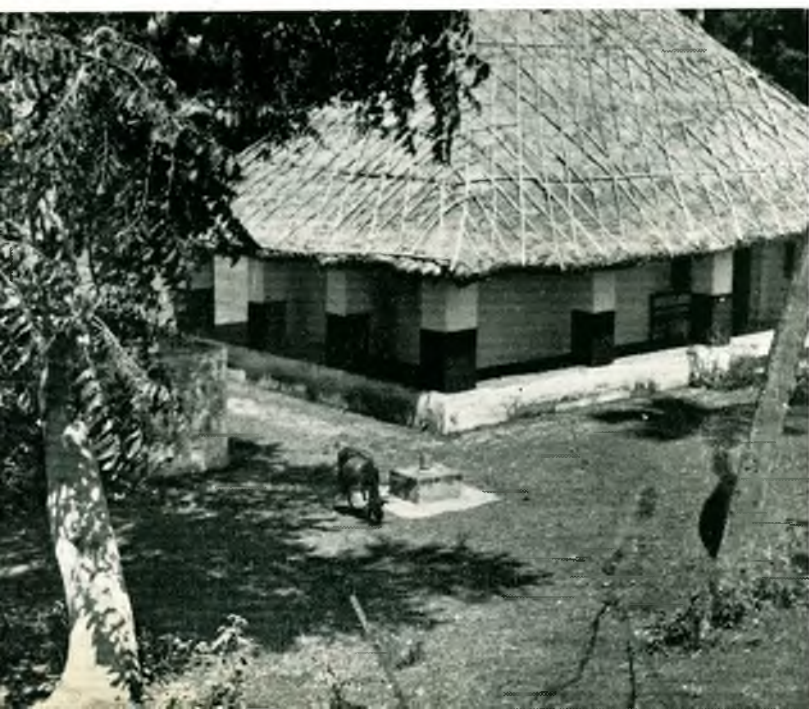
Ext. C/99 (2) Mahal tree, rain gauge, urinal and firing position of P. S. thatch in south-west corner
