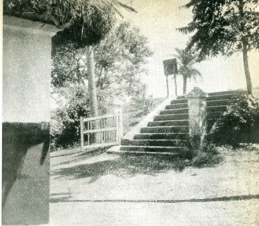
Ext. C/99 (5) Gate and steps of P S, embankment road, south- west corner pillar and thatch of the P. S.
