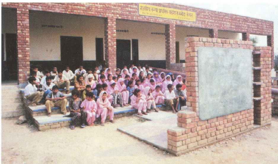
An amphitheatre made by widening the existing steps up to the plinth, with a stage and chalkboard in front.
