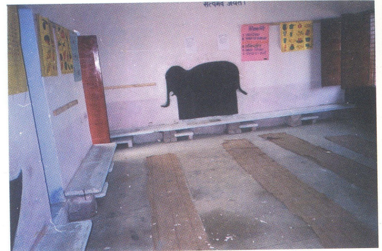
Here ferrocement benches have been placed all along the classroom walls. Storage spaces are provided underneath.
