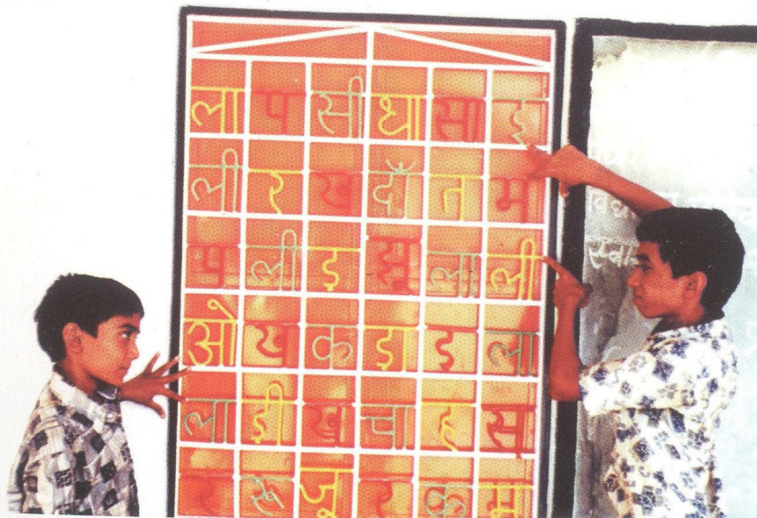
* The window grill becomes an interesting learning aid. Care should be taken in design of grills that those which face the outside may be used only from inside, while those facing the verandah may be used from both sides.
