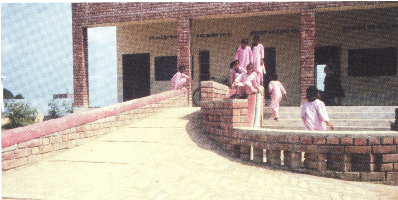
An attractive ramp has been provided here and is the main entrance for all.
