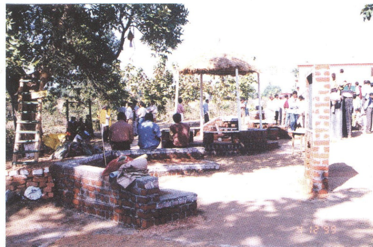
**Low cost external 'classrooms' in Mandla distt., MP. the amphitheatre seats are in the shade of a tree, and face a chalkboard. A circular set of benches has a low cost roof as a shade.
