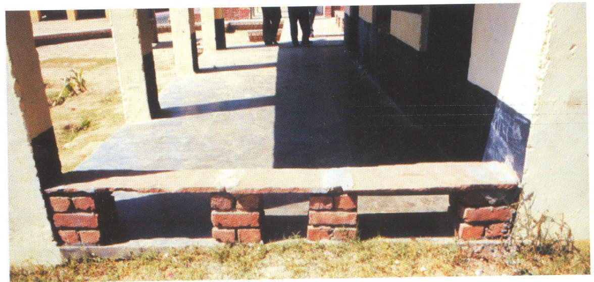
Benches can be provided in the verandahs too.
