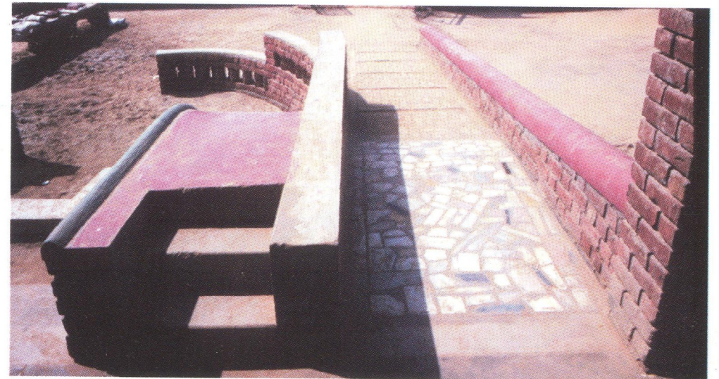
Steps up to the slide from the verandah. The side wall of the ramp is shared with the slide.
