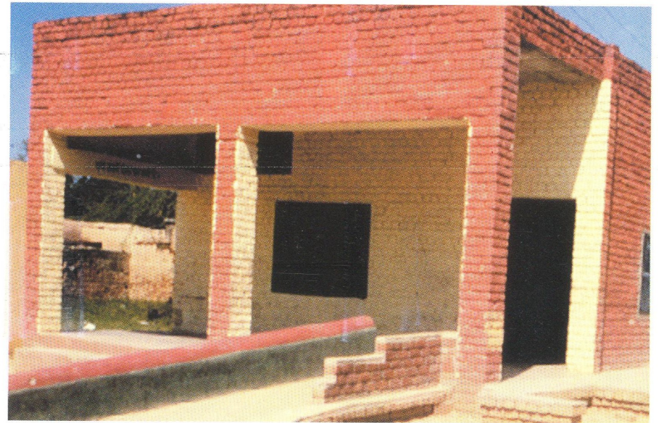
A verandah, which costs about 80% of a classroom.
