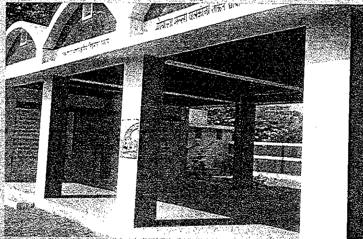
Block Resource Centre in Aurangabad, Maharashtra Constructed by the Centre for Science in Villages, the BRC provides large semi-covered spaces. Cost effective systems of construction have been adopted. This includes the use of guna tile roofing and unburnt mud bricks for the walls.
