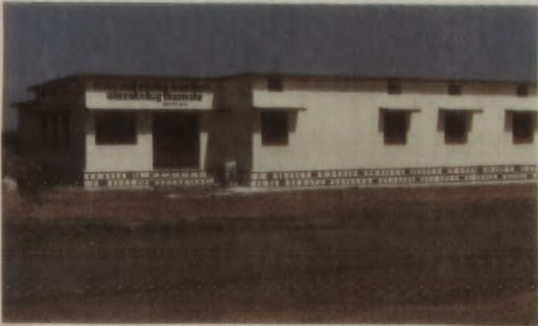
BLOCK RESOURCE CENTRE BUILDING
