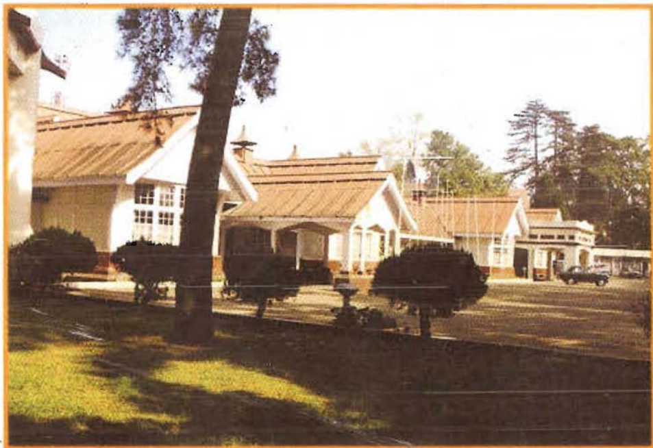
Meghalaya Legislative Assembly, Building Structure - 1912 to 9 th January, 2001
