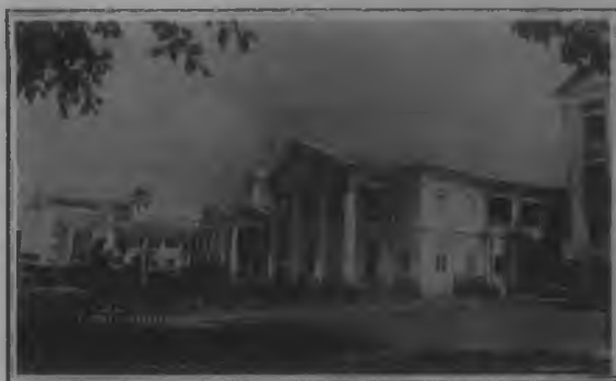
The Kerala Govt. Secretariat building - the seat of the State administration. This imposing building in the lines of Roman-Dutch architecture, was built during the reign of H.H. Ayilyam Thirunal Rama Varma, Maharaja of Travancore (1860 - 1880)
