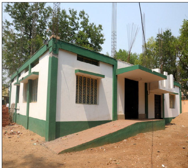
Construction of Minority Bhaban at Suri.
