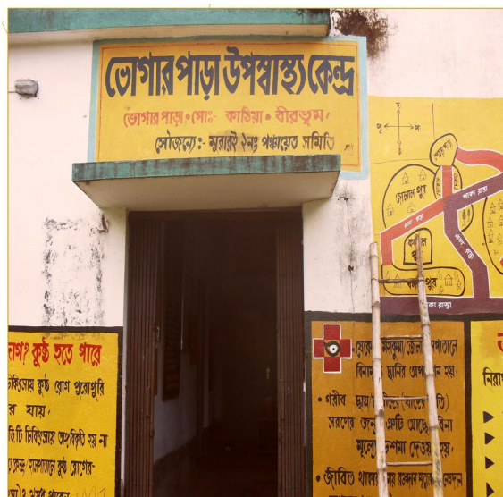
Health Sub-Centre at Murari-II Block
