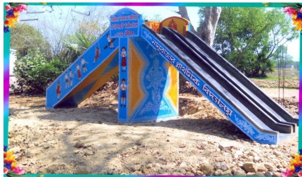
Construction of Child Friendly Element
