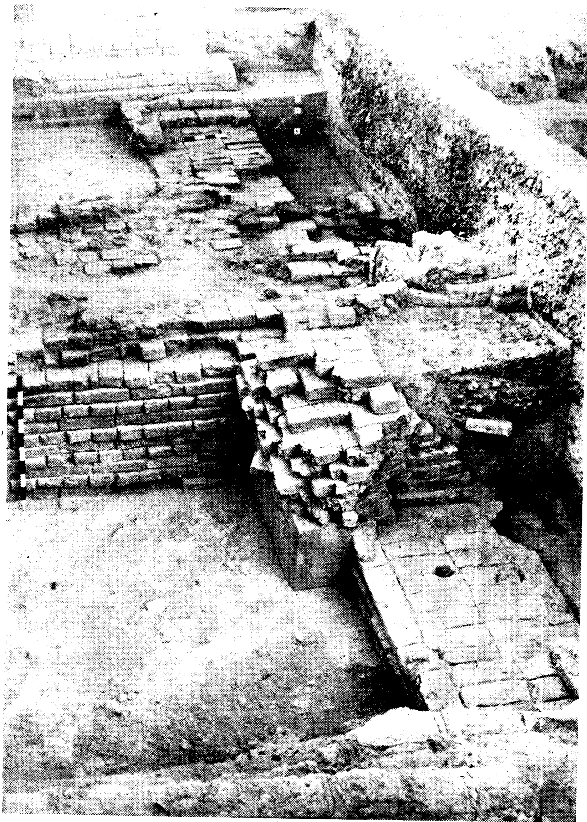
Banawali : Passage of the Harappan Gate and Drain
