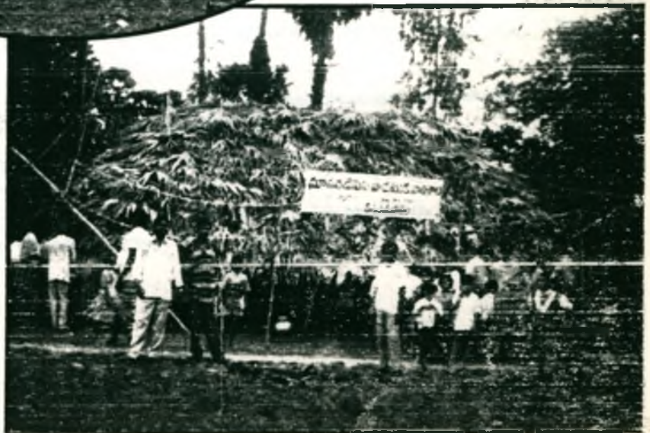
Temporary thatched Shed for locating New DPEP School built by the Villagers at Kasireddipalem
