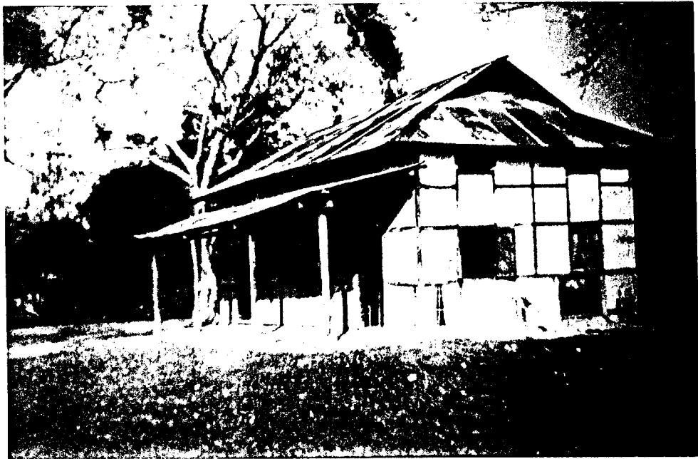
Barigaon L.P. school. Udalguri, Darrang.
