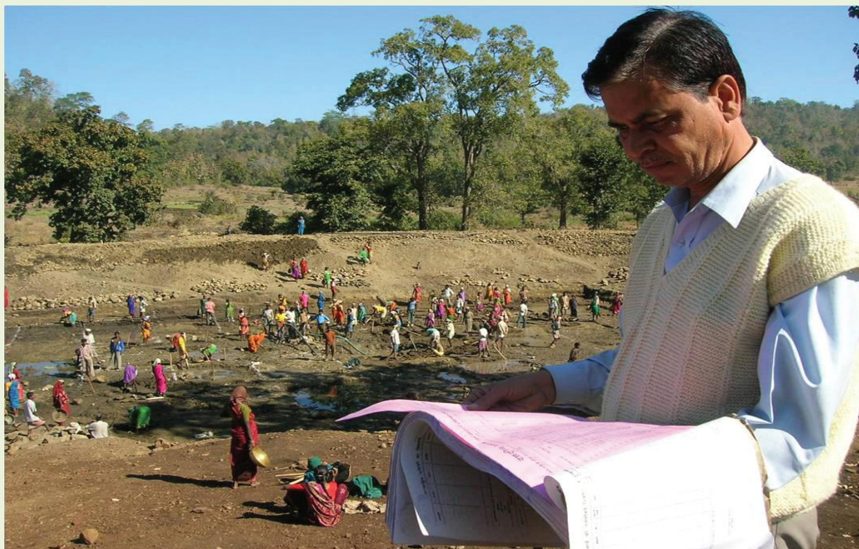
MGNREGA work in progress
