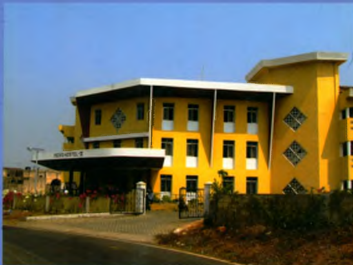
A glimpse of the new Boys' Hostel Block at the Goa University campus.
