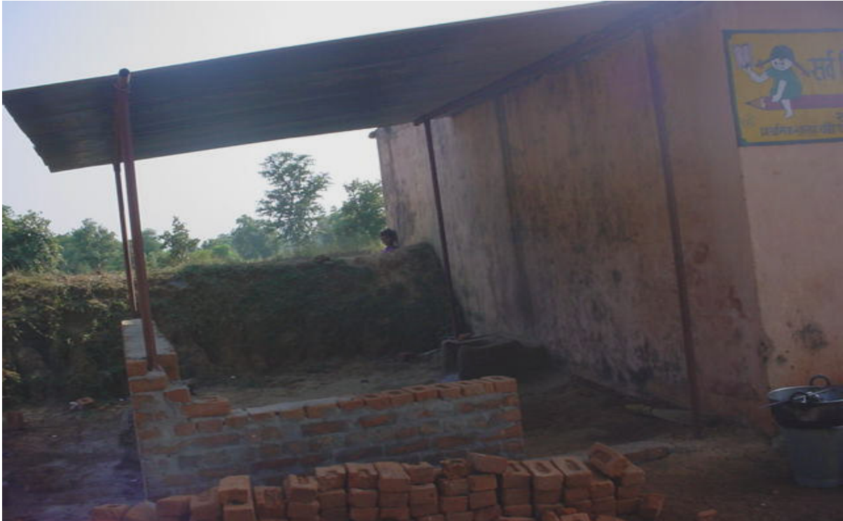
Community support in construction of kitchen shed
