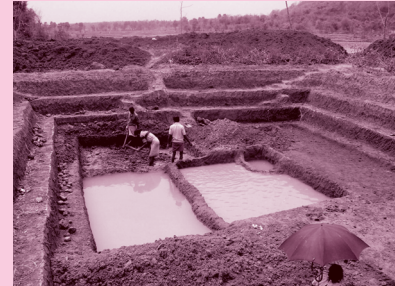
2.5.4 Construction of 5 percent model going on
