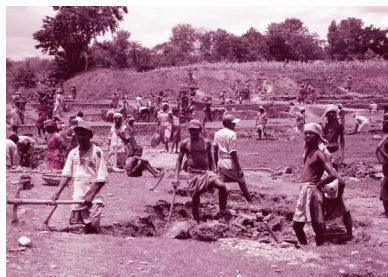
6.4 Work under NREGP going on
