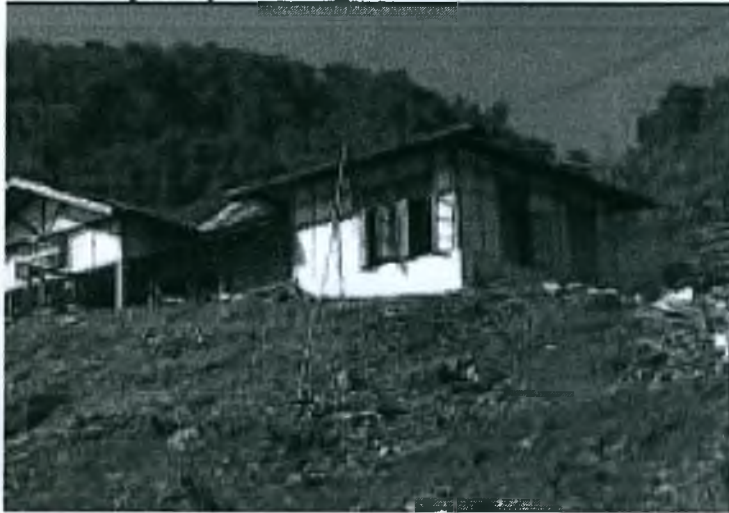
Anchal Samity Hall used for hostel accommodation
