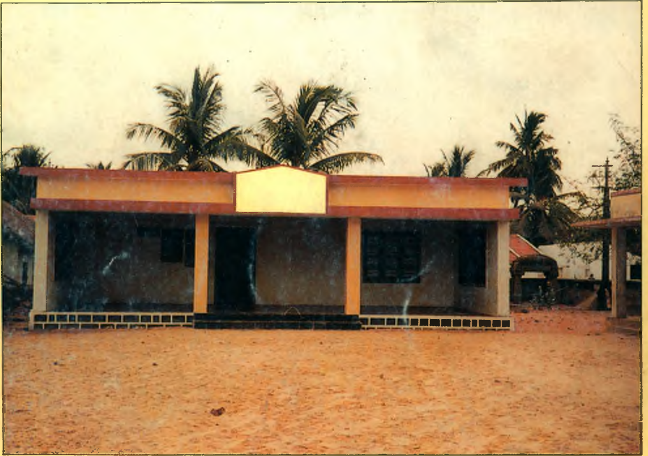
A TEACHERS' CENTRE BUILDING
