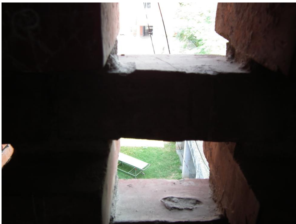
PGI INN WINDOWS IN GMHS- SECTOR-12 BUILDING
