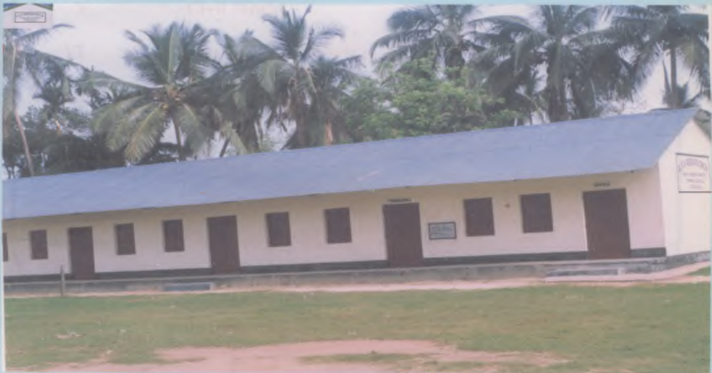
PHOTOGRAPH OF BRC BUILDING CONSTRUCTED AT CHOWDHURI BARI GIRLS H.S. SCHOOL FOR JIRANIA BLOCK
