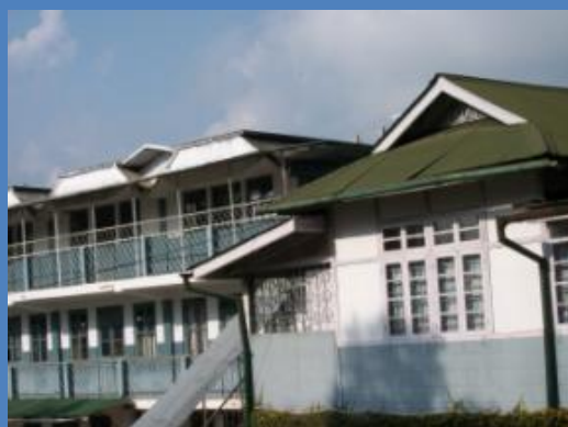
School Building of Shullai Progressive School
