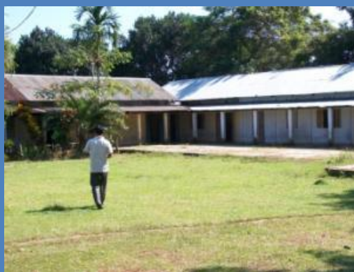
School Building of Karukol U.P. School
