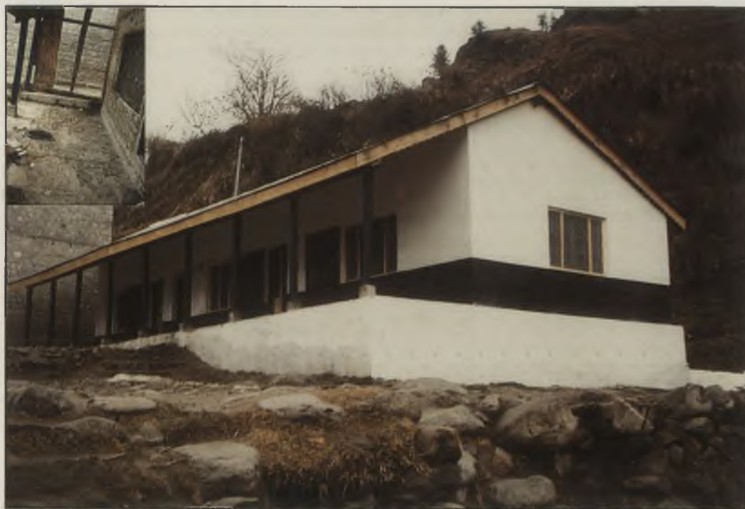
School building before repairs (inset) and after repairs - Himachal Pradesh.
