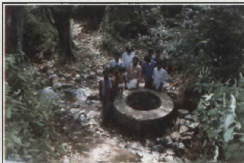
An open well dug for drinking water near the school. The top circular structure is constructed with locally available laterite stones
