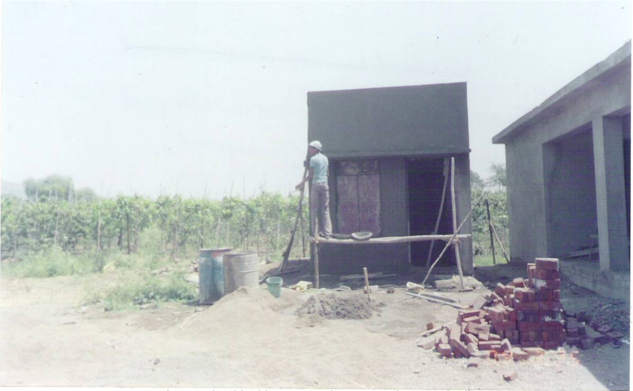
Construction of new school building at Finishing stage (Aurangabad)
