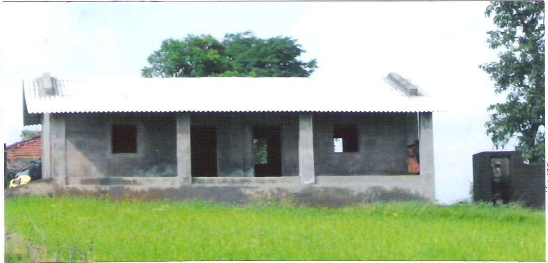
Completed New school building with Toilet facility
