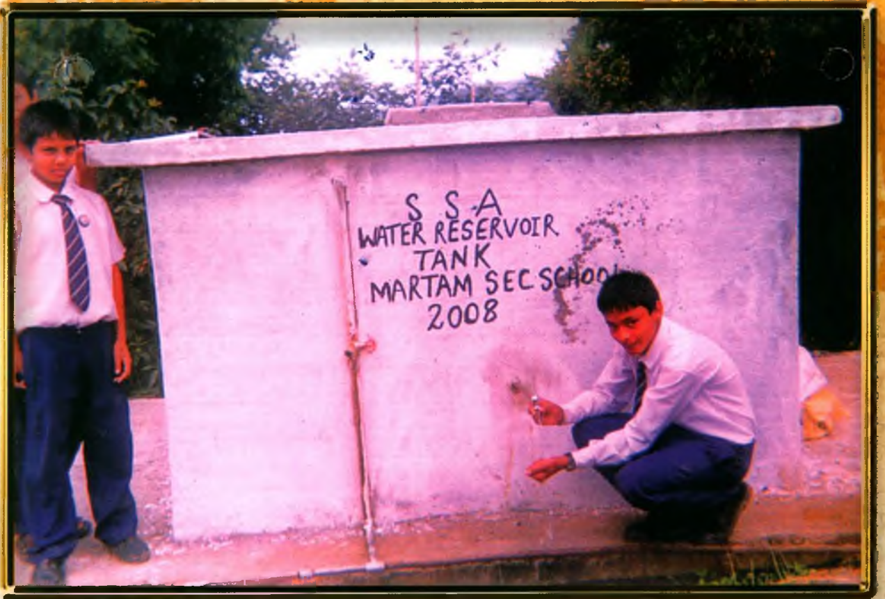
S.S.A. Water Reservoir Tank (Martam Sec-School - 2008)
