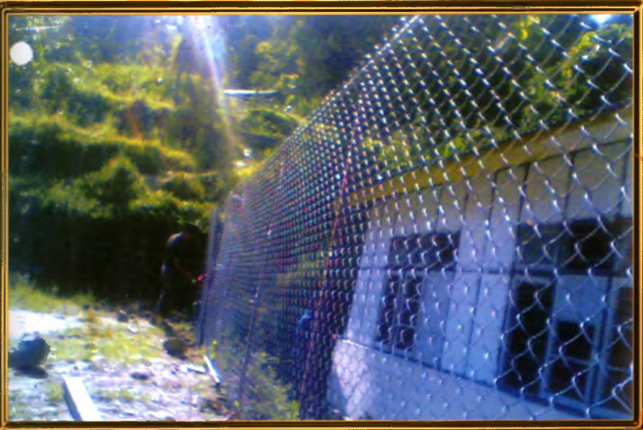
Boundary Wall (Sang - Tshalamthang Jr. High School - East Sikkim)
