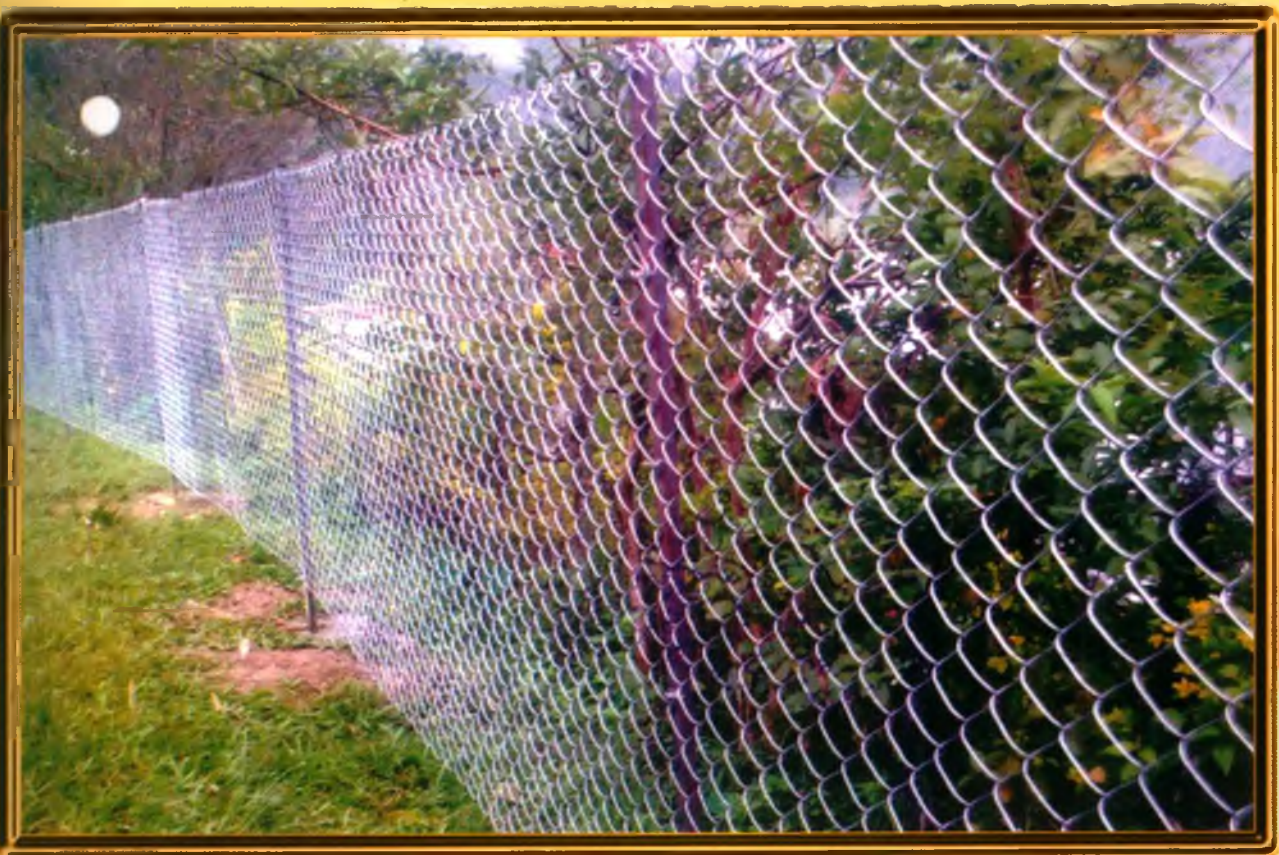
Boundary wall under S.S.A. (Sang Chalamthang J.H.S. (East))
