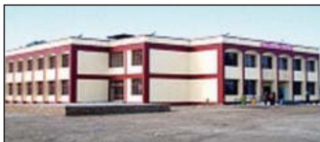
New Upgraded (under RMSA) Govt. Secondary School Building, Punjab.
