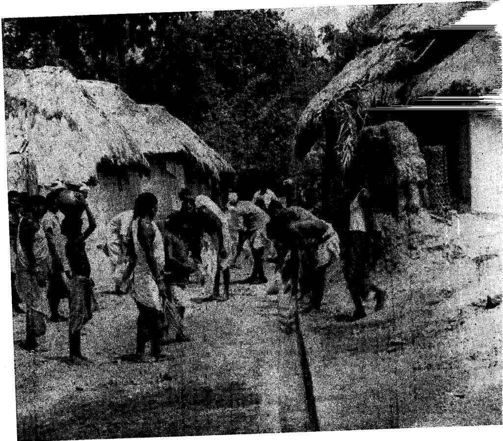
A cemented drain being erected in an Adivasi village of Dumka.
