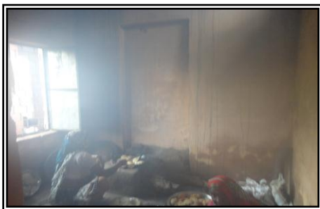
Kitchen filled with smoke
