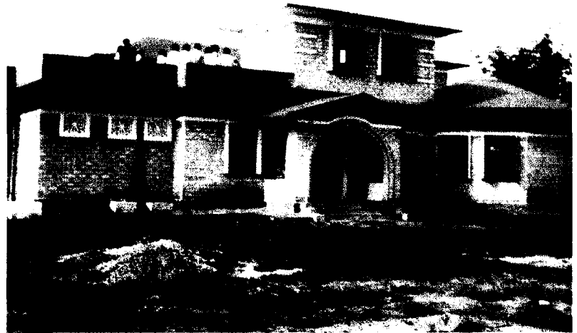
Rat-trap bond wall and filler slab roof used in BRC construction of Bihar - cost savings of 20 - 24 % without compromising on the quality and aesthetics of the building
