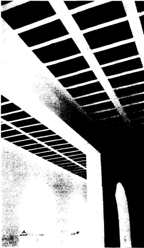
School construction in Karnataka - use of cost-effective Filler Slab roof
