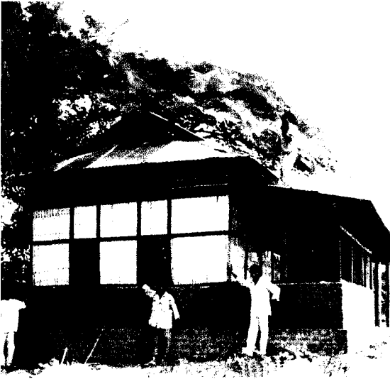
Bamboocrete walls and CGI sheet roofing in Assam - use of traditional technology
